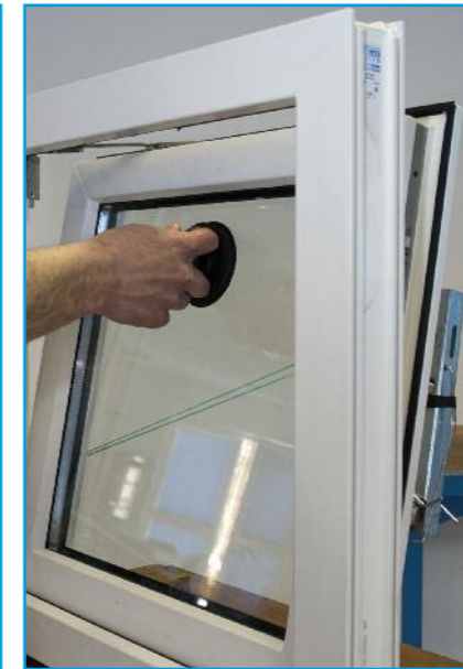
Pull traction rope over bolting system. Pull traction rope diagonally downwards and close window.
